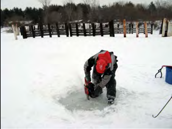
Cutting Ice Block Out Of Ice Sheet
