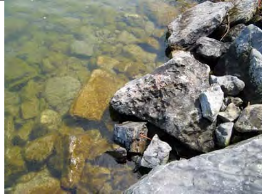
Marked Rip-rap (#1): May 4, 2009
