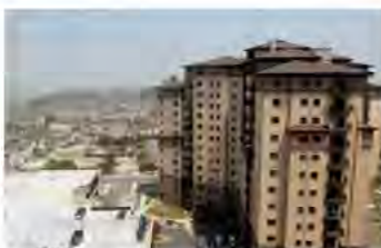
New family housing constructed at Osan AB, Korea
