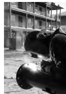
New dorm under construction at Keesler AFB, MS
