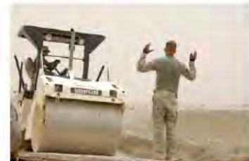
RED HORSE team uses heavy construction equipment
