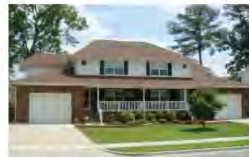
Military Family Housing at Seymour Johnson AFB, NC
