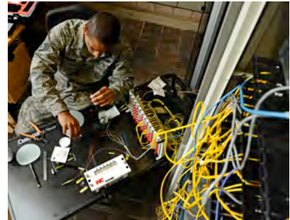
Air Force NCO repairs optical fiber cable
