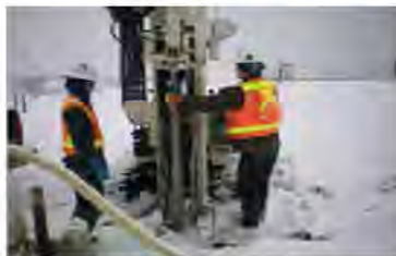
Monitoring Well installation at former Galena FOL in Galena, AK
