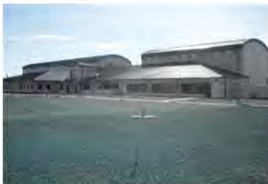
Recently completed state-of-the-art training complex for the Inter American Air Forces Academy at Joint Base San Antonio, TX
