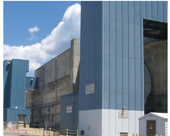
The interior of the building resembles a canyon because the processing areas resemble a gorge in a deep valley between steeply vertical cliffs. The canyon facility's walls are 835 feet long, 122 feet wide and 66 feet high.
