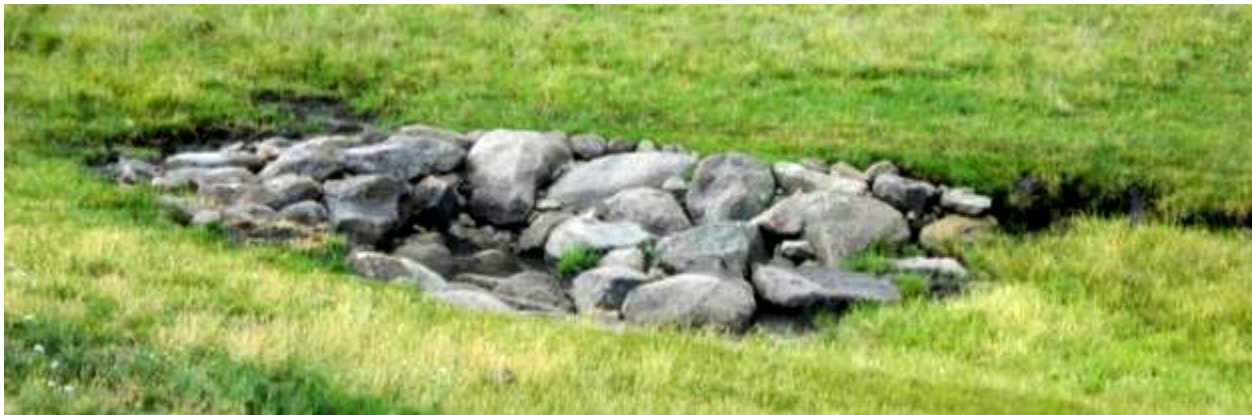
Figure 4 – “Zuni Bowl” constructed in the Valle Santa Rosa.
