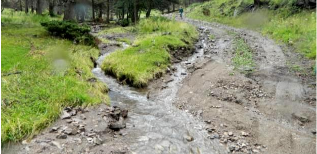
Figure 3 – Road VC-13, post fire erosion
