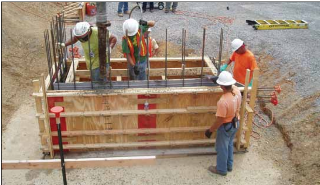
Workers construct a concrete sump at Cell 6
