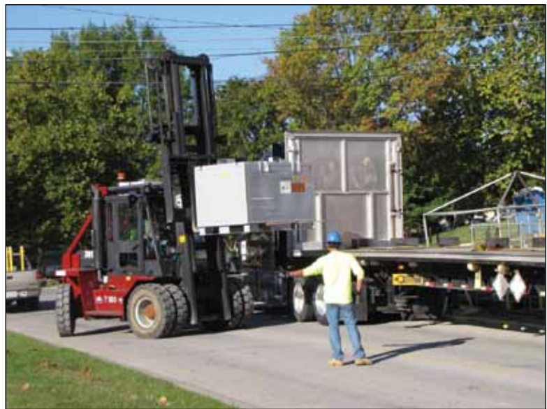
Contaminated soil from Tank W-1A excavation is being shipped to the Nevada National Security Site for disposition.
