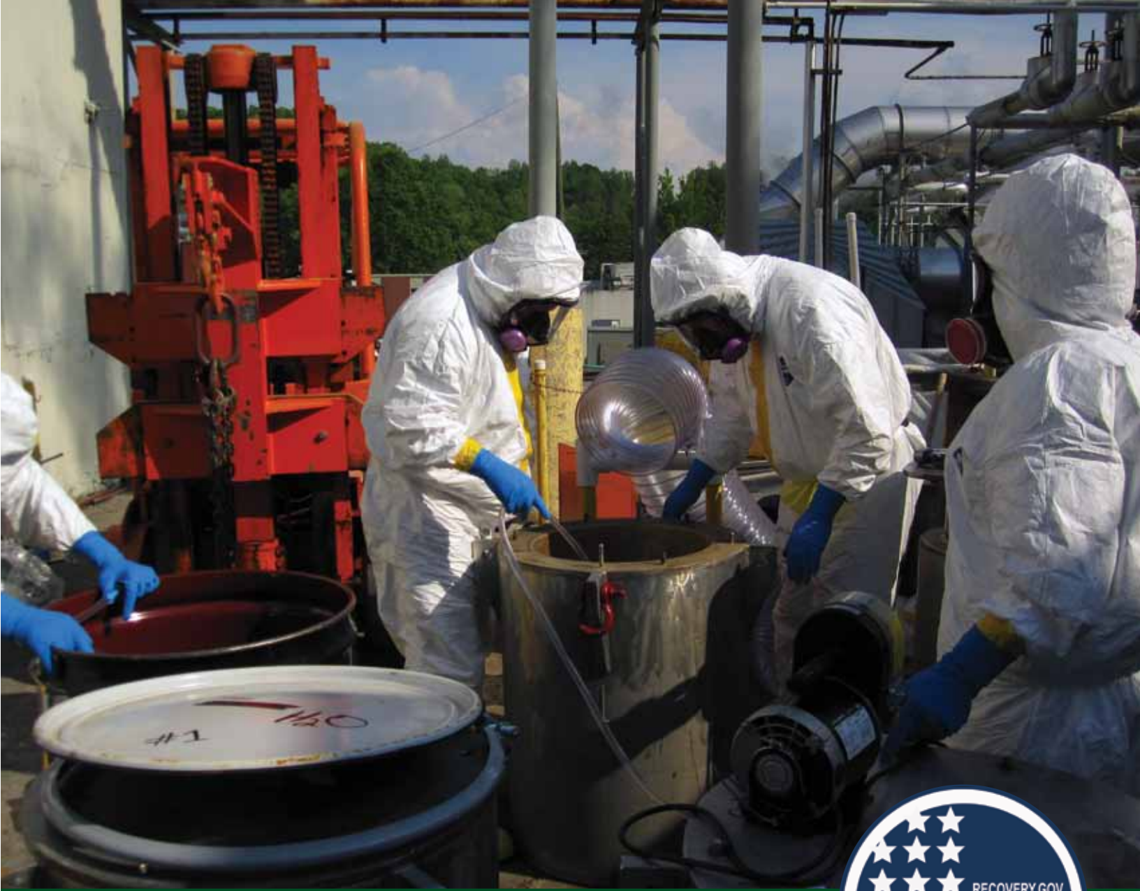
Workers inspect a shielded carrier used for disposal of Isotope Row legacy material.
