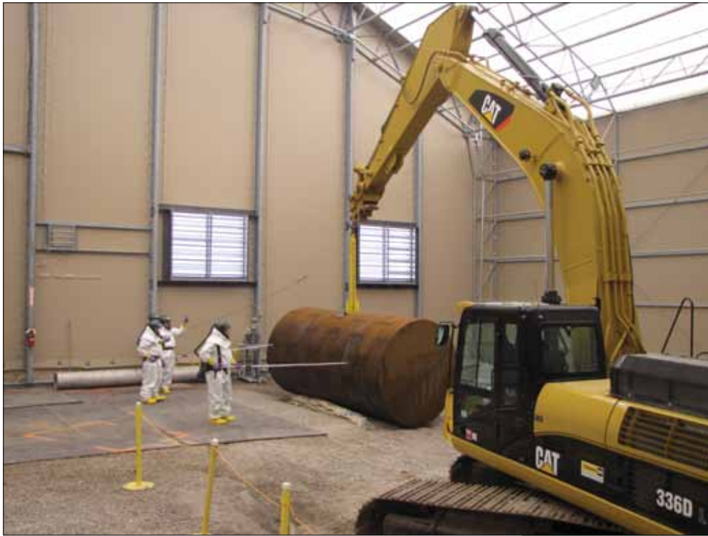
Workers practice tank removal inside the Tank W-1A enclosure.
