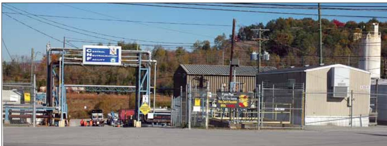
Central Neutralization Facility
