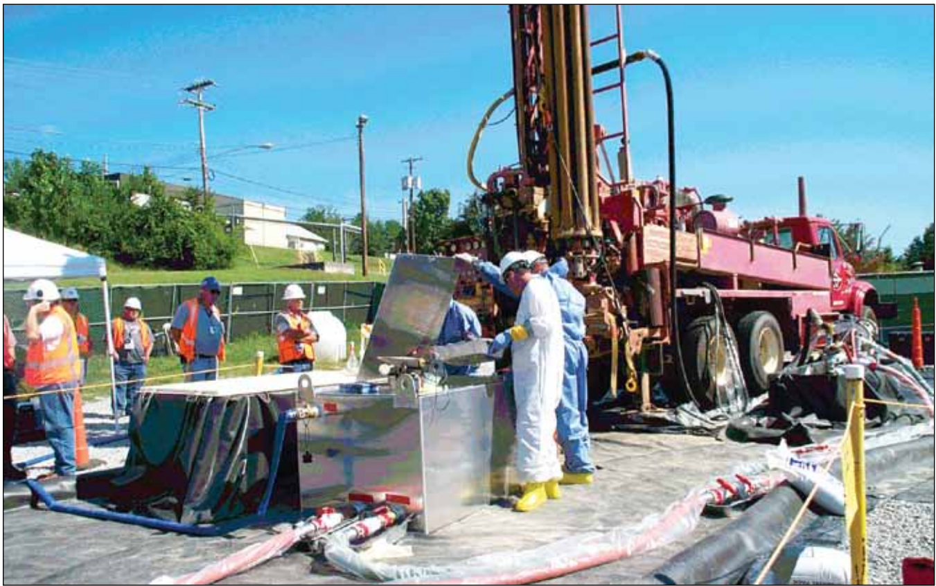
Corehole 8 extraction well drilling
