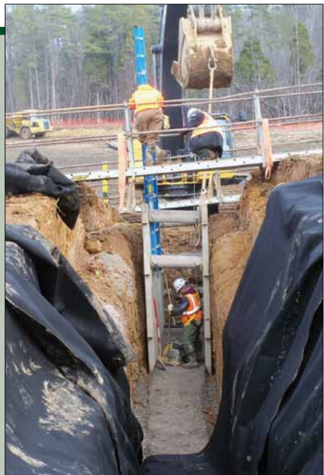
Workers install a French drain at SWSA 3 to divert shallow groundwater and rain water away from the capped areas.
