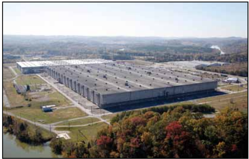
K-33 Building before demolition
