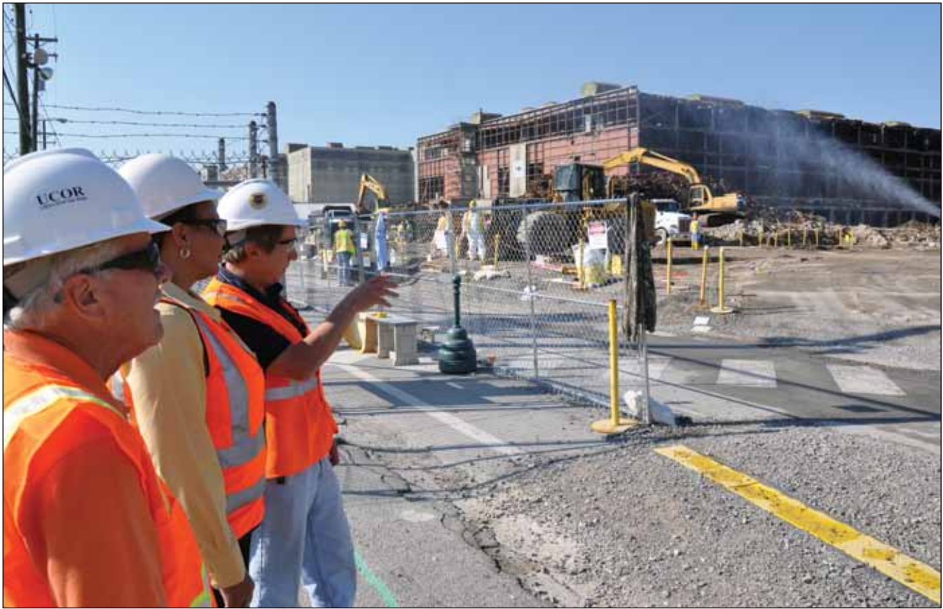
K-25 Project Manager Mark Ferri, right, discusses the K-25 Building east wing demolition with UCOR President and Project Manager Leo Sain and ESH&QA Manager Cheryl Cabbil.
