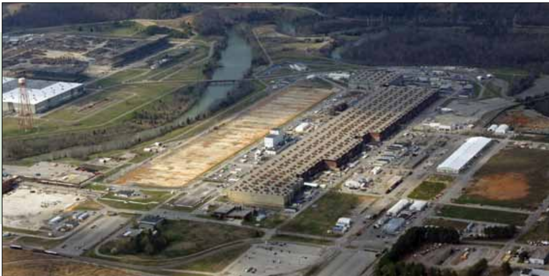
East wing before demolition began; the west wing was previously demolished.
