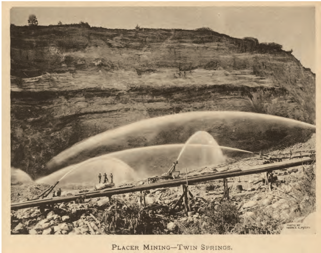
Figure 4.3. Mining was an important part of Idaho history particularly in northern Idaho (Silver Valley), central Idaho (Elk City), and the Boise Basin. Placer mining, Twin Springs, Idaho (published 1901). Photograph obtained from Library of Congress, Prints and Photographs Division, Horace C. Myers, [reproduction number: LC-DIG-ppmsca-17299].
