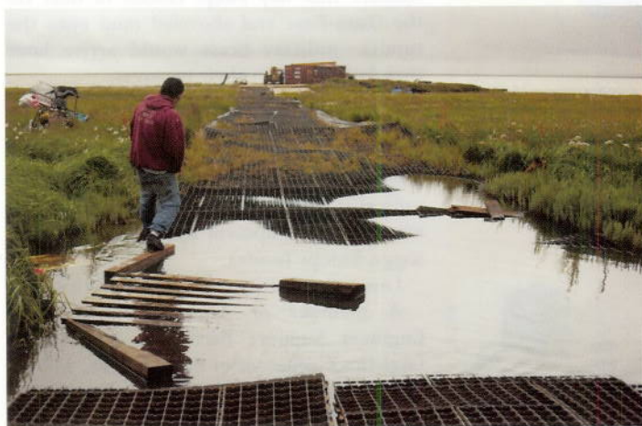
The walkway to the barge landing site in Newtok is formed by loose wood planks and mats.
