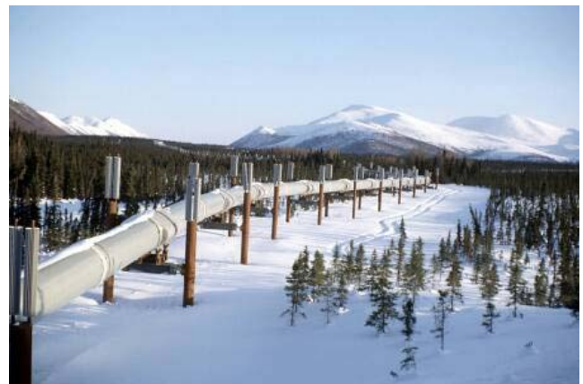
The TAPS includes both buried pipe and pipe supported on steel structure above ground, depending on local soil and geologic conditions.
