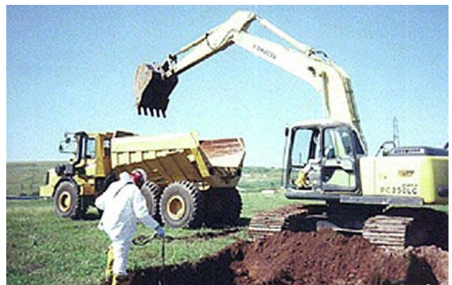
Application of precision excavation at the Ashland 2 FUSRAP
