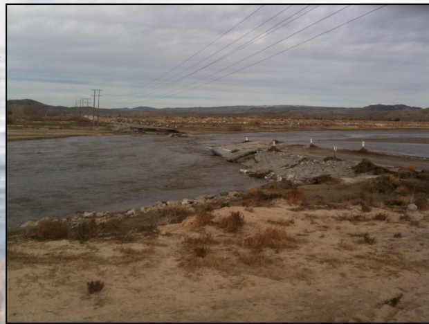
The Mojave River washed out a bridge at Lenwood in December 2012 due to flooding from heavy rain, and snow in the mountains. (Photo: John Fertsch)
