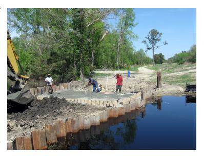
geosynthetic gravel-filled cells has been used as a facing to provide erosion protection to the GRS abutments. Despite construction delays on the project due to preloading and differential settlement, traditional construction would still have been more expansive and time consuming. Technology applied on this project supported the FHWA EDC initiative.
