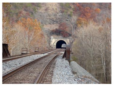
greater than 21' above the top of the rail. In addition to the tunnel work, there are 29 other overhead obstructions that need to be removed or adjusted. These additional obstructions include: 8 bridge replacements; 8 bridge removals; 4 bridge raises; 2 bridge modifications; and 7 track modifications.
