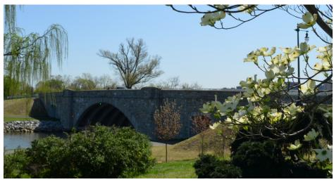
The replacement of the historic Humpback Bridge was designed to incorporate all existing architectural features (including reuse of all existing stone) into the replacement structure. The grade of the road adjusted was improve sight distance over the bridge. A pedestrian crosswalk was replaced with a
