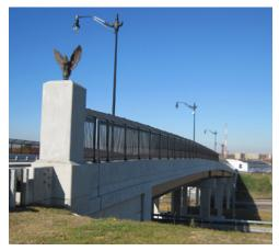
This Design-Build project involved the design and reconstruction of the 9th Street Bridge over New York Avenue, NE, and connecting roadways. The new bridge replaces a 70 year old bridge over railroad tracks for the CSX and Metro. It features wider lanes and sidewalks to provide space to bicyclists, as the city is experiencing a welcome boom in bike traffic.
