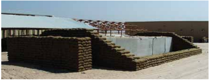
Semi-hardened bunker, without collective protection.
