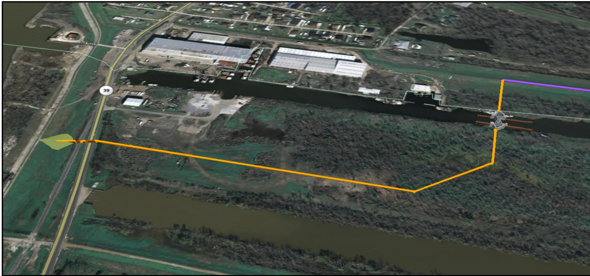
Figure 2.4. Aerial view of the Caernarvon Floodwall and Gate in St. Bernard and Plaquemines Parishes.
