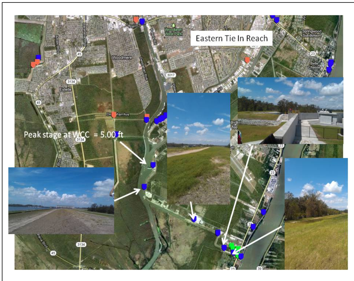
Figure 4.17 Damage assessment team data from the Eastern Tie-In Reach.
