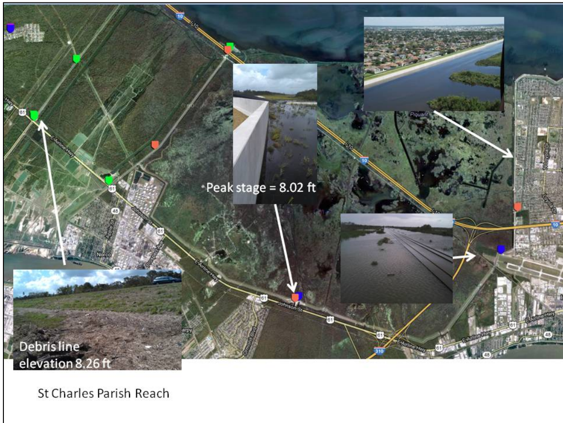
Figure 4.14 Damage assessment data from the St. Charles Parish Reach.
