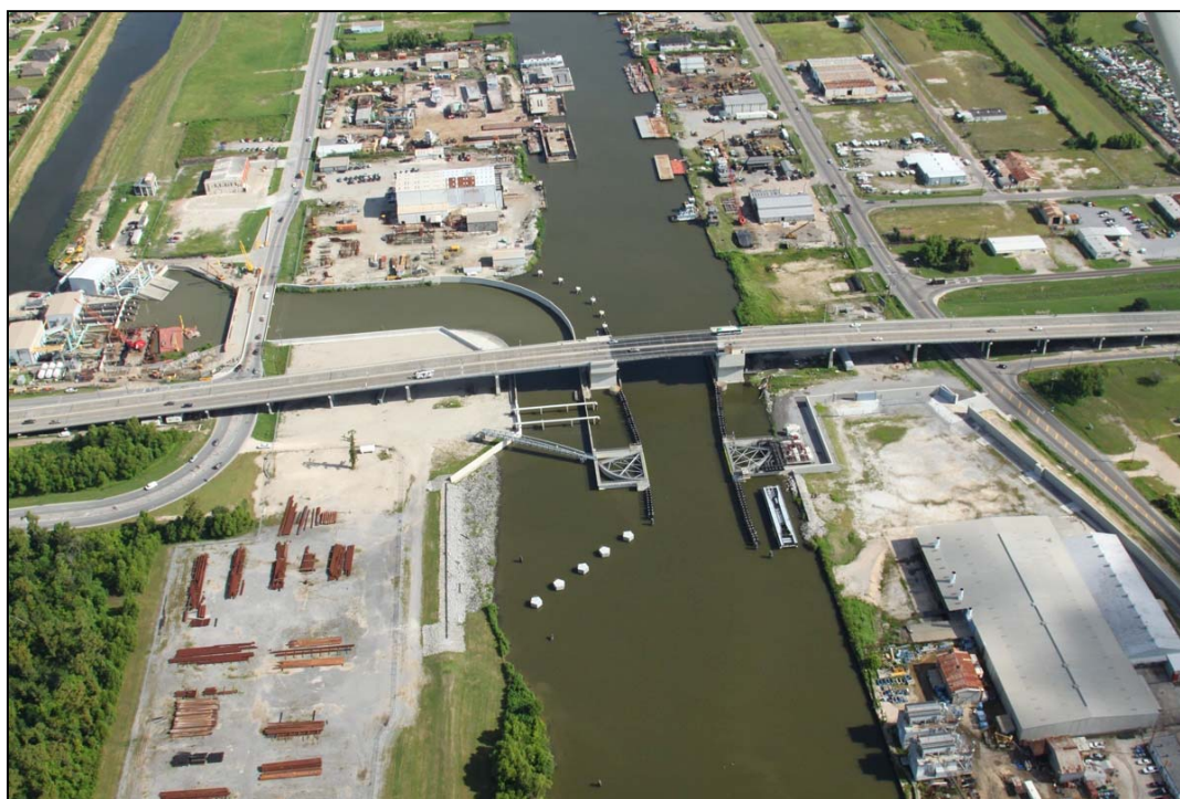
Figure 2.7 Aerial view of the Harvey Sector Gate on the Westbank in Jefferson Parish.
