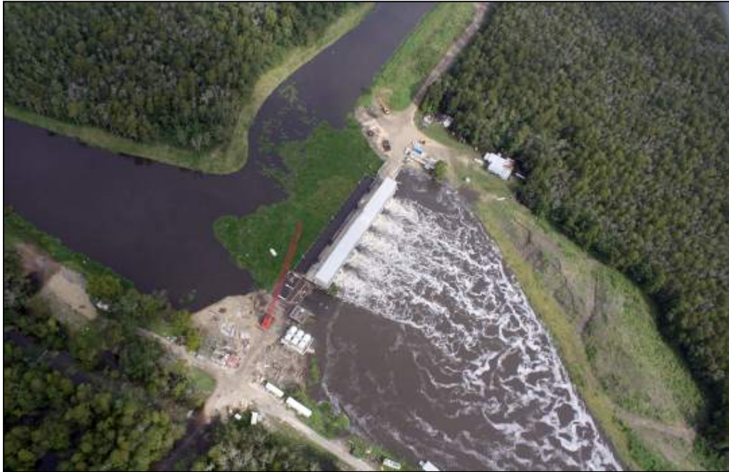
Figure 7.3.11 Aerial image of Marvin J. Braud Pump Station in Ascension Parish during normal operations.
