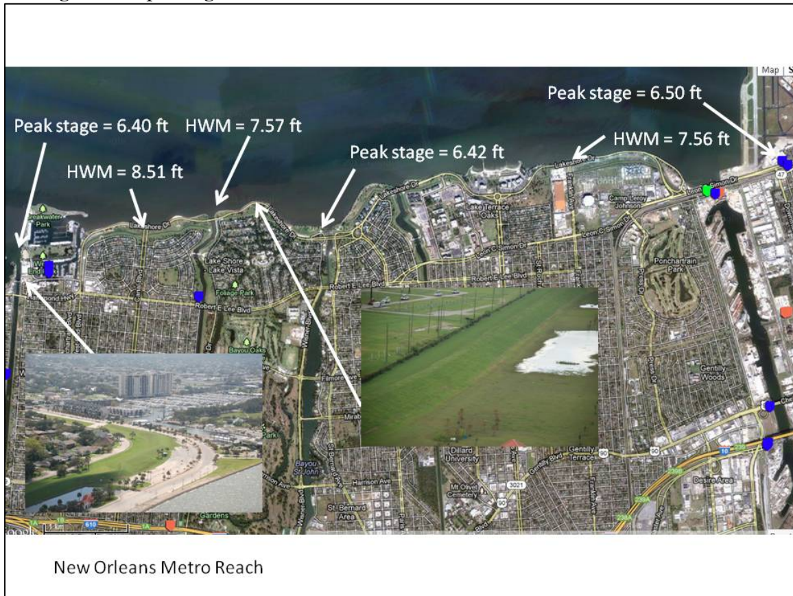
Figure 4.12 Damage assessment data from the New Orleans Metro Reach. High water mark data courtesy of South Louisiana Flood Protection Authority-East.
