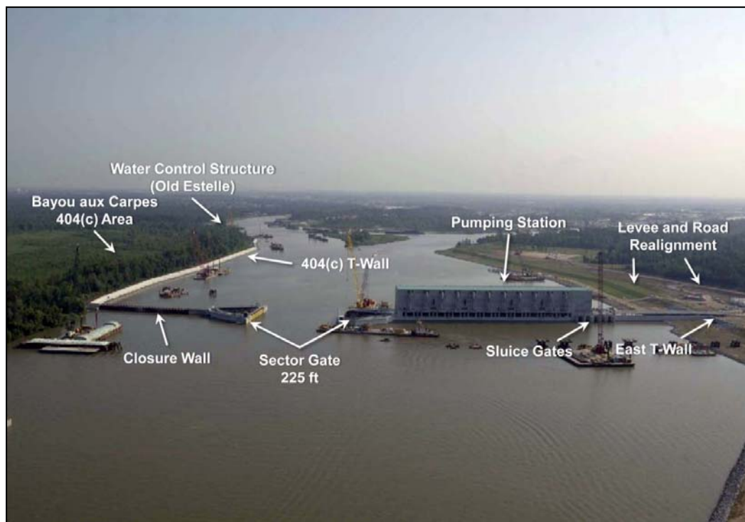
Figure 2.6. Aerial view of the West Closure Complex and Estelle Water Control Structure in Plaquemines and Jefferson Parishes.
