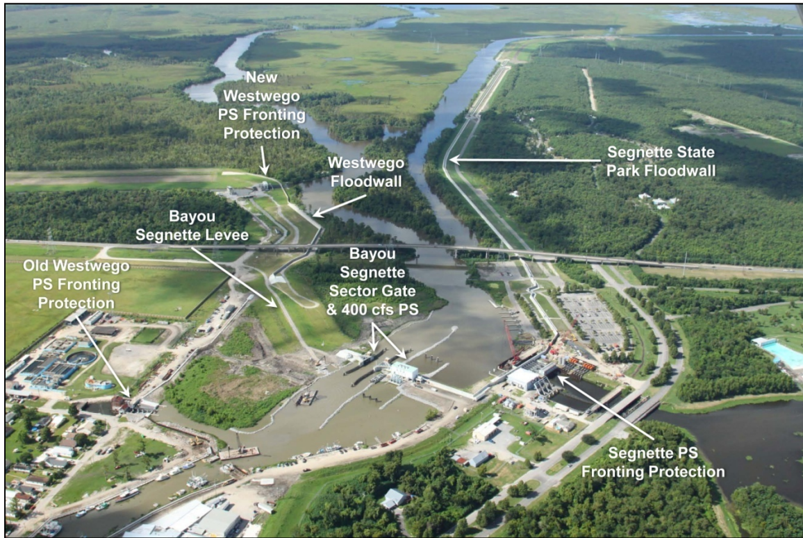
Figure 2.8. Aerial view of the Bayou Segnette Complex on the Westbank in Jefferson Parish.
