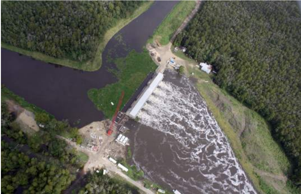
Figure C-10 Aerial image of Marvin J. Braud Pump Station in Ascension Parish during normal operations.
