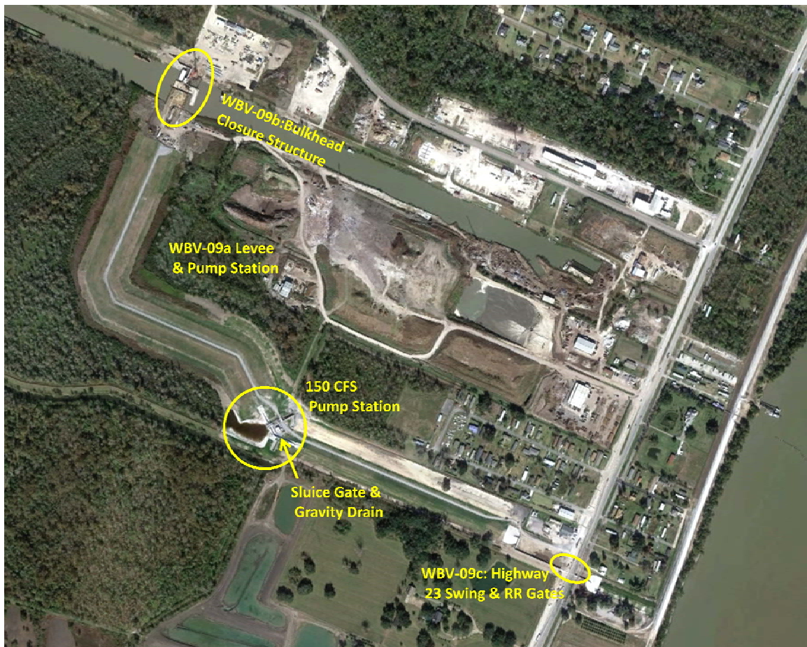
Figure 2.5. Aerial view of the Eastern Tie-In projects on the Westbank in Plaquemines Parish.
