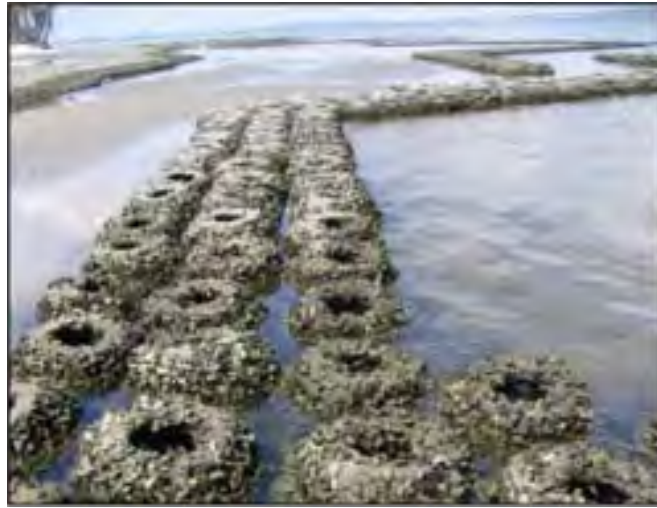
Figure 2-23: Oyster Reef Alternative - Interlocking Concrete Rings
