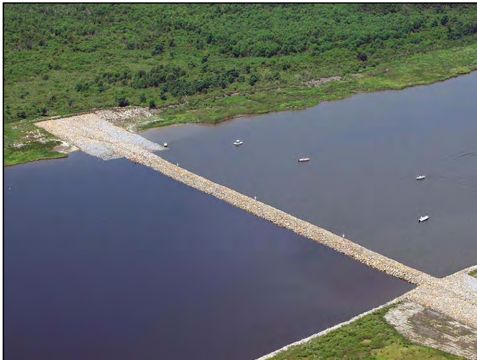
Figure 1-4: MRGO Closure Structure at Bayou La Loutre
