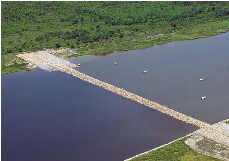
Figure 3-1: MRGO Closure Structure at Bayou La Loutre Completed July, 2009
