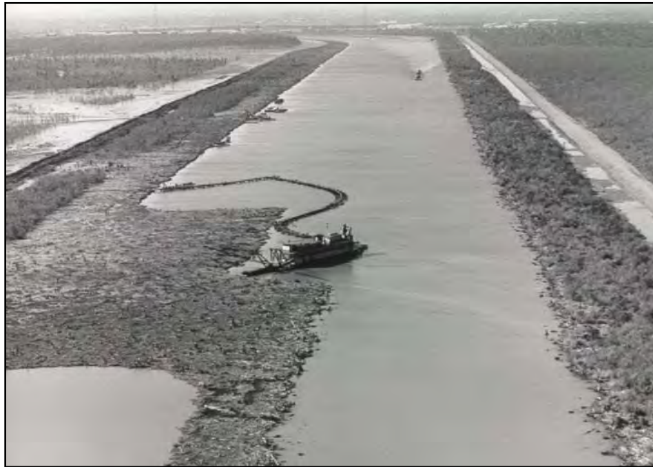
Figure 1-5: Construction of MRGO Channel (1959)
