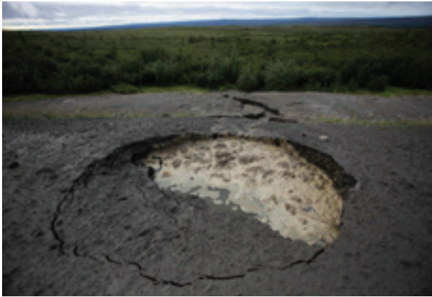
Permafrost melt resulting from global warming is damaging infrastructure across the Arctic. This section of the Dempster Highway in Canada's Northwest Territories collapsed because of thawing permafrost.
