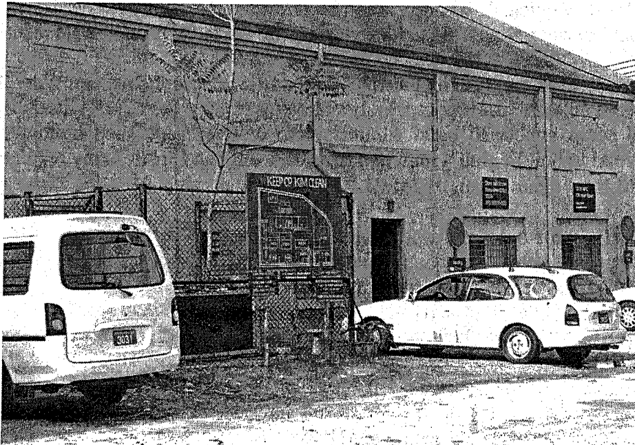
Camp Kim, One of the Former Japanese Warehouses.
