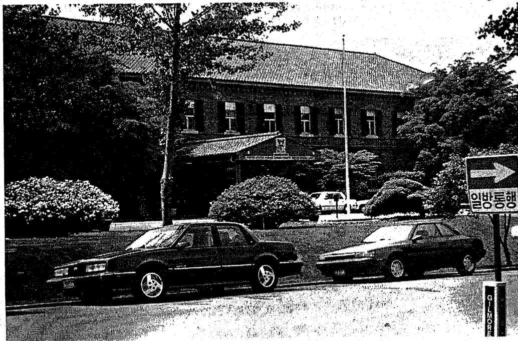
Hodes Hall, Former Japanese Barracks
