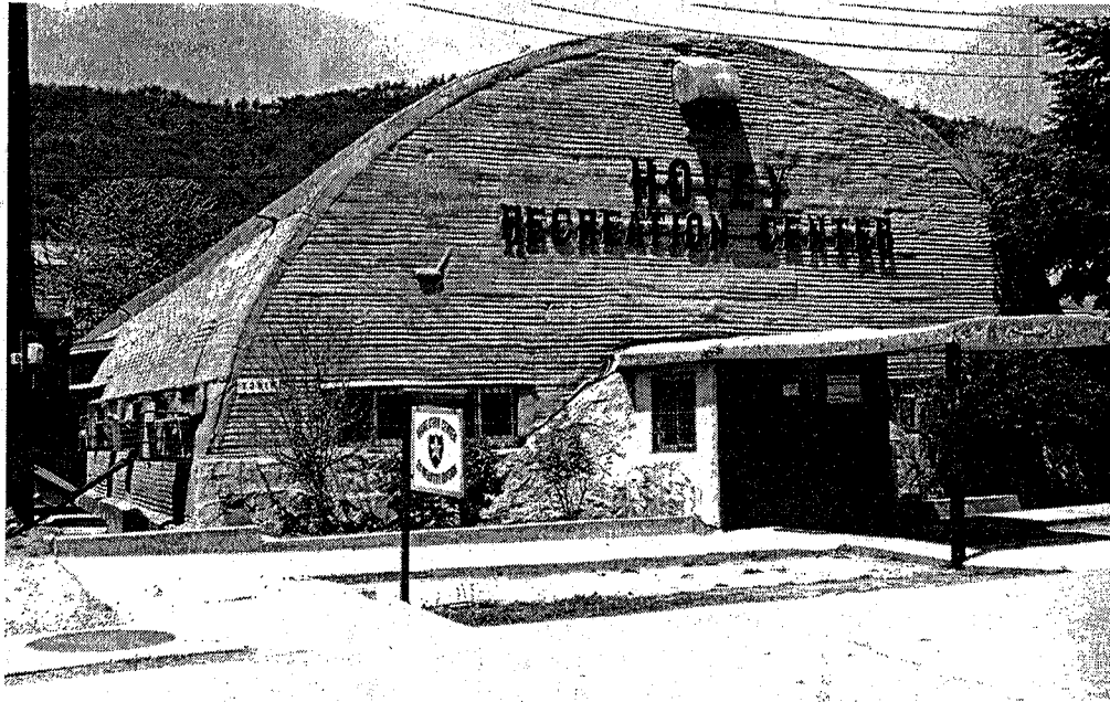
Hovey Recreation Center in Elephant Quonset Hut.
