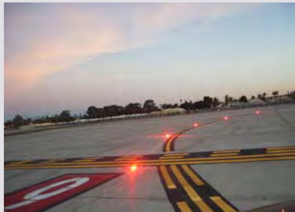
RWSLs are used to hold takeoffs, as well as to signal when aircraft may or may not enter a runway.
