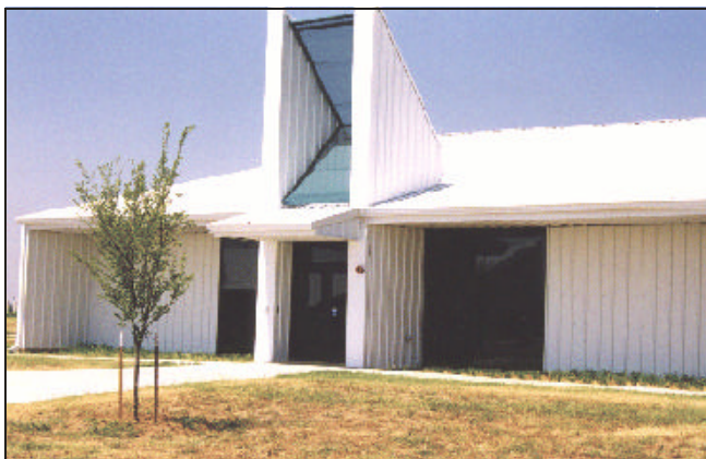
New landing system training building at the Mike Monroney Aeronautical Center
