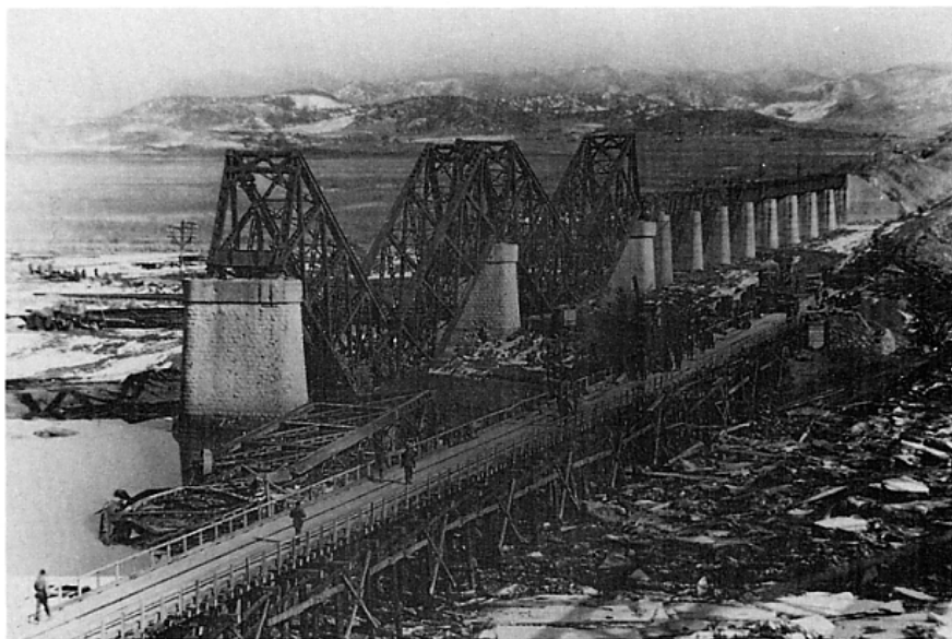
Figure 7. The low-level pile bridge at the Freedom Gate site that the 84th Engineer Construction Battalion erected in January–February 1952 between two destroyed railway spans. The shadow cast by the more southerly of the railway bridges, which the 84th would reopen in July 1952, is visible at the right of this 10 March 1952 photo.
