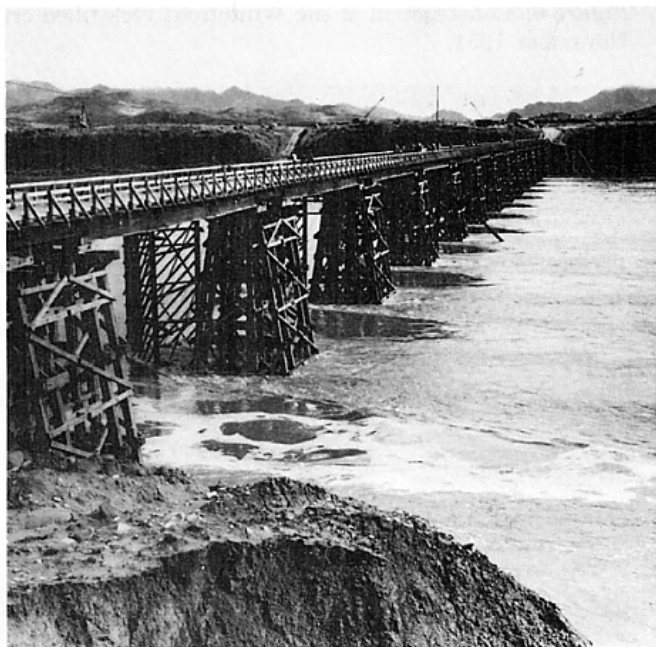
Figure 7. The low-level pile bridge at the Freedom Gate site that the 84th Engineer Construction Battalion erected in January–February 1952 between two destroyed railway spans. The shadow cast by the more southerly of the railway bridges, which the 84th would reopen in July 1952, is visible at the right of this 10 March 1952 photo.
