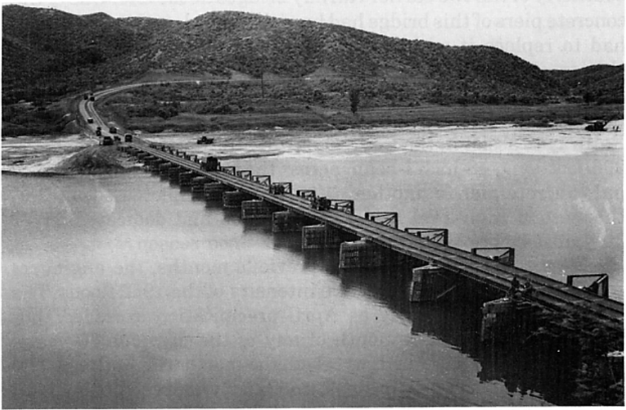
Figure 17. Spoonbill bridge on 20 June 1953.
