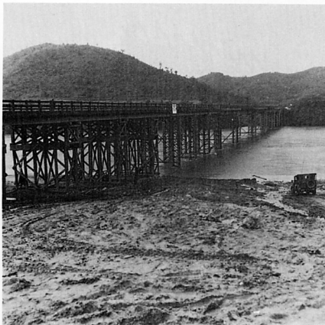
Figure 10. The high-level White-front bridge on 27 July 1952.
