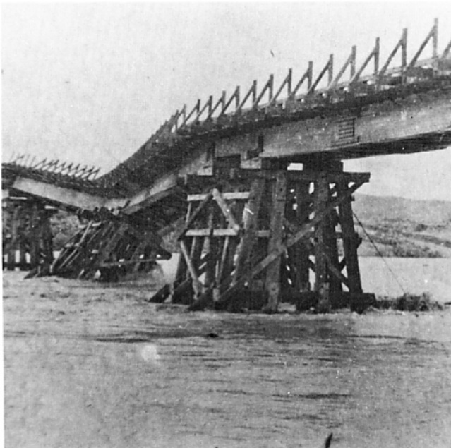
Figure 12. The high-level Teal bridge collapsing under the pressure of floodwater on 30 July 1952.
