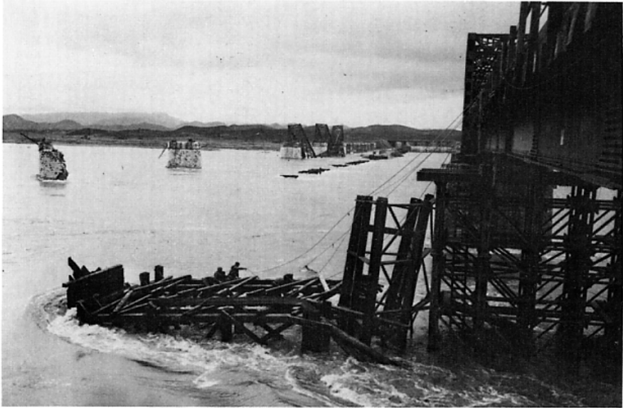
Figure 13. Pier from the collapsed high-level Teal bridge lodged against protective fender piles at the reopened span of the Freedom Gate bridge on 30 July 1952.
