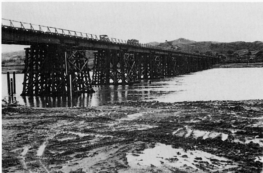
Figure 9. The high-level Pintail bridge on 27 July 1952, just three days after the 62d Engineer Construction Battalion had opened it.
