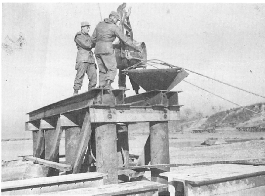
Figure 24. Troops filling the hollow Armco piles with concrete, with 36-inch I-beam girders in the foreground.
