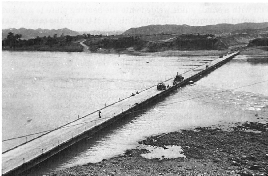
Figure 37. Teal bridge after the flood of 15 July 1953 showing the damage to the removable guardrail, which was not removed due to the rapid rise of the river.
