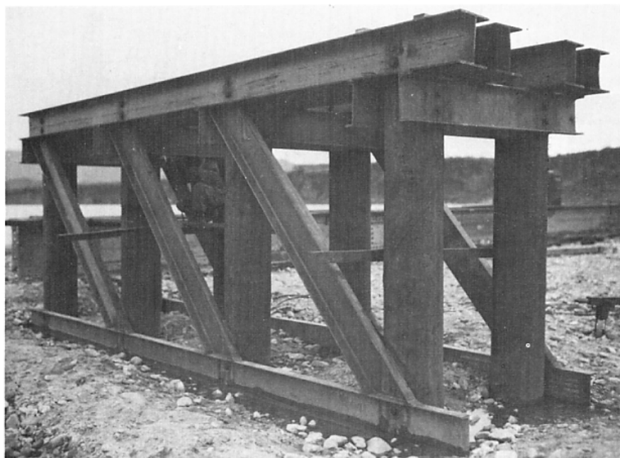
Figure 22. A nearly completed pier featuring diagonal channel-iron bracing.
