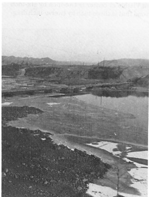
Figure 31. Teal bridge from the south shore on 7 January 1953 as troops place decking on the north end.
