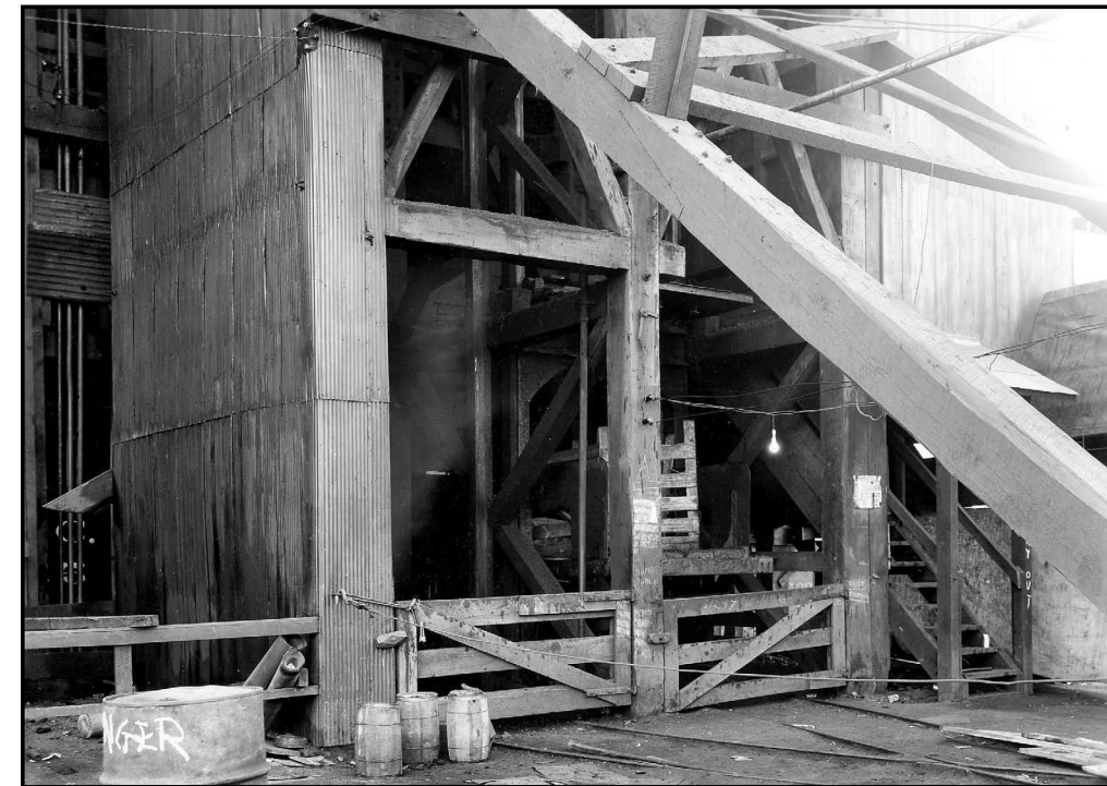
Sunday Creek Coal Company – Surface landing of the main shaft. Photo Bureau of Mines
