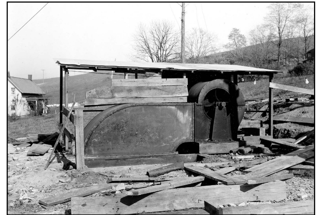
Sunday Creek Coal Company – Fan, new air shaft. Photo Bureau of Mines
