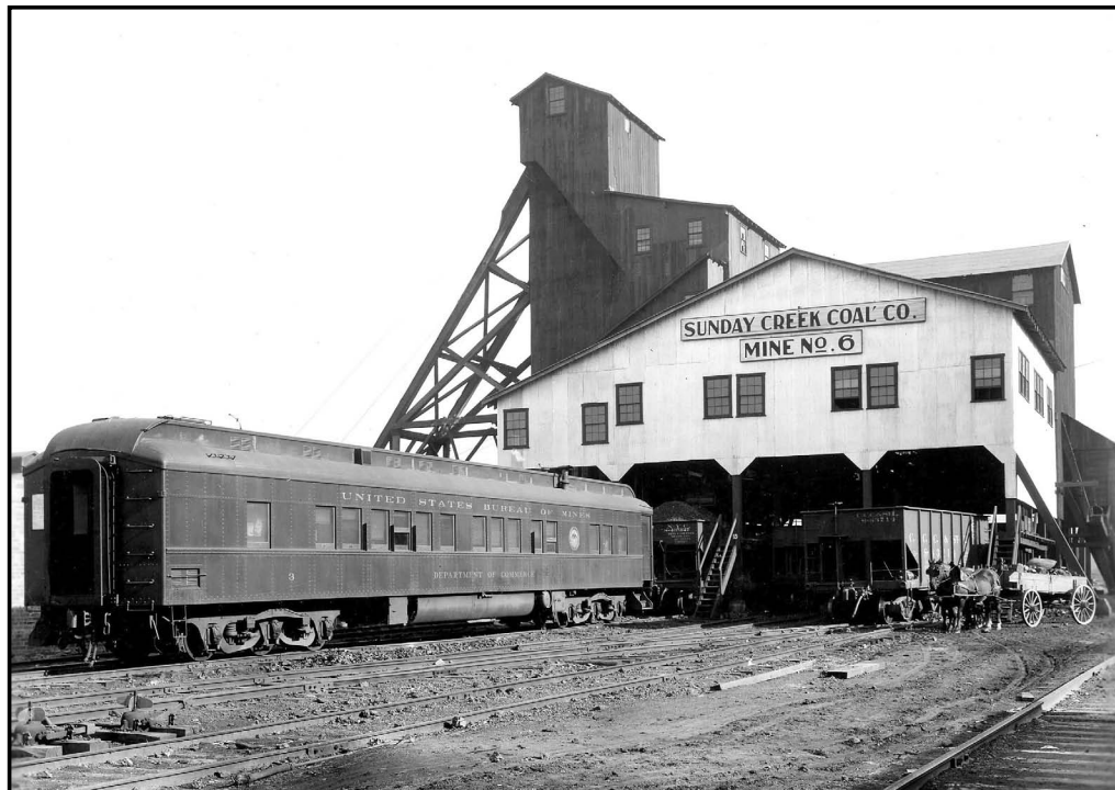
Sunday Creek Coal Company – Tipple, loading dock and Mine Safety Car No. 3. Photo Bureau of Mines
