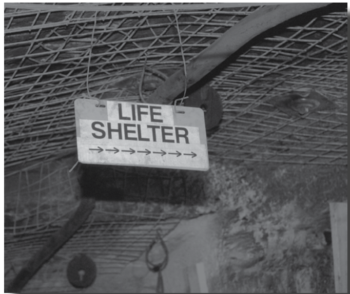
Sign pointing to a Refuge Chamber.
