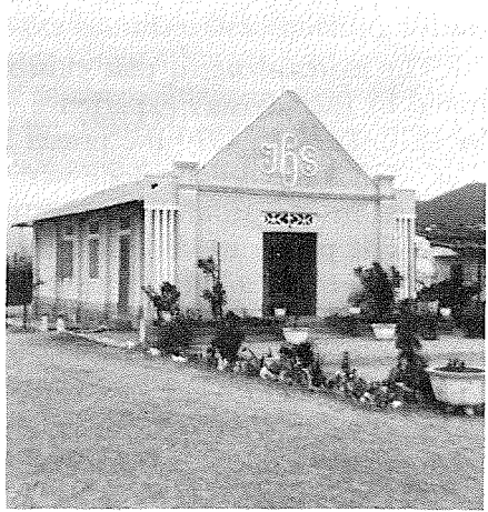
CHAPEL OF THE MILITARY PRISON AT DANANG. Judge advocates helped to procure building materials.
