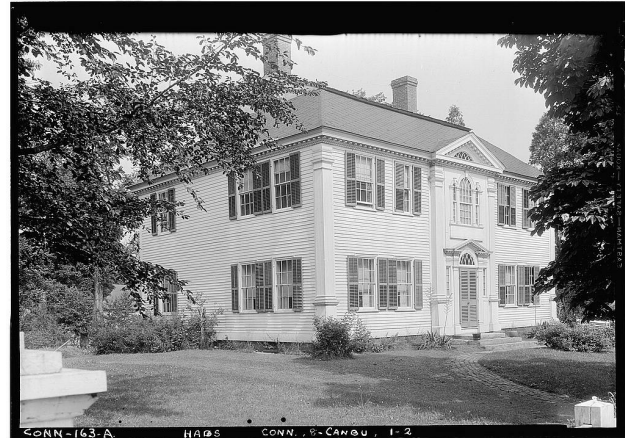
Figure 11 Elisha Payne House/Prudence Crandall School, Canterbury, Connecticut. This house was built in 1805 for an Elisha Payne born later than the one on the Sheep Census. Prudence Crandall bought it in 1831 and established her school there. The photograph was taken on July 16 1940 by the Historic American Buildings Survey. Photographer: Stanley P. Mixon. Prints and Photographs Division, Library of Congress, Washington DC. HABS Conn, 8 - Canbu, 1-2. View online .
