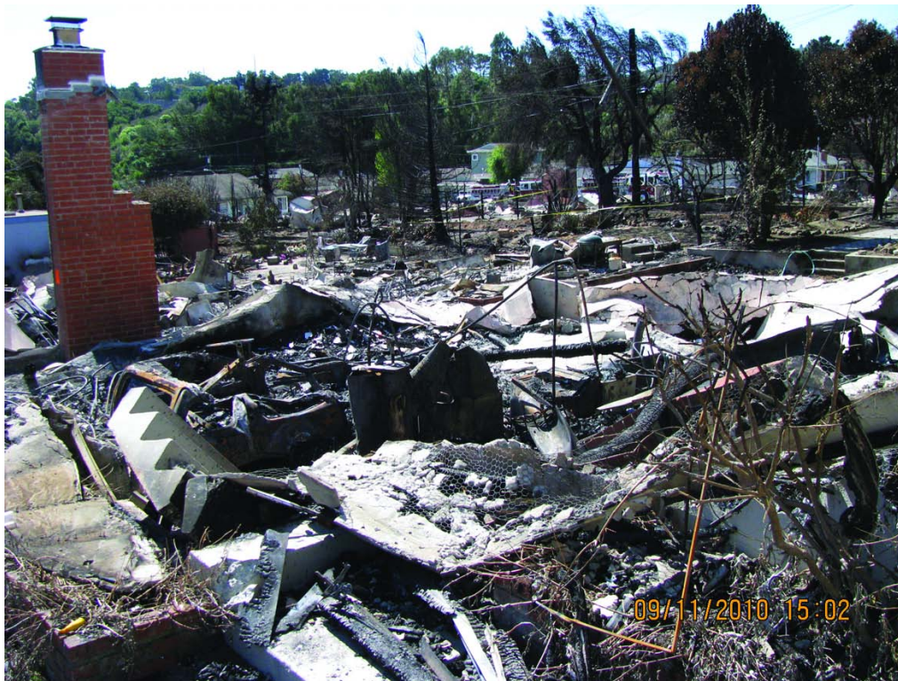
Figure 12. Picture of destroyed houses.
