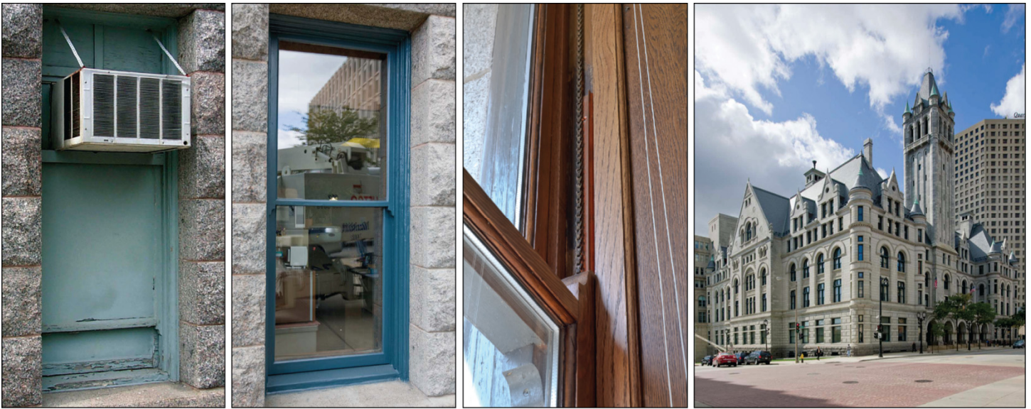
Figure 1: Milwaukee Federal Building and Courthouse Window Repair
