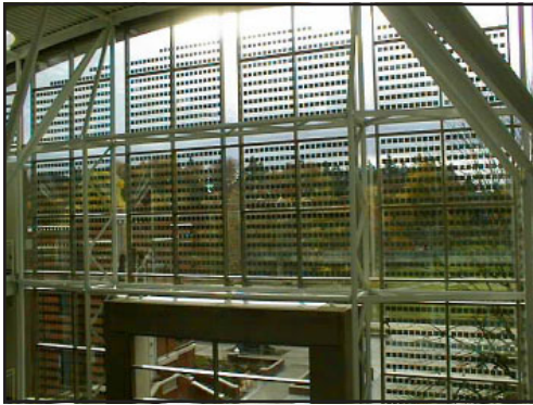
Figure 11 — University of Oregon's Lillis building shows PV cells integrated into vertical glass.
