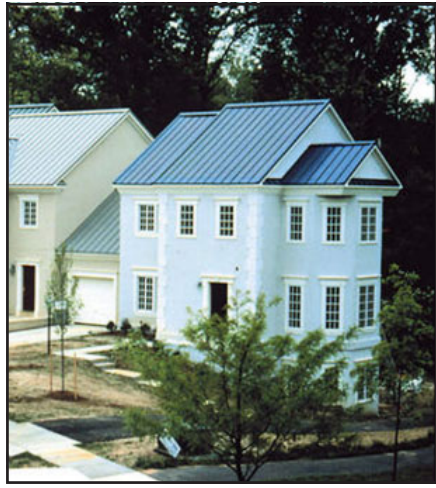
Figure 12 — Roof integrated thin-film modules
