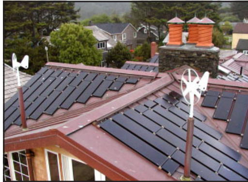
Figure 6 — East- and west-facing collectors are okay if the roof slope is not too steep.
