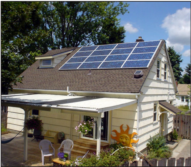
Figure 1 — Solar powered 1929 home in Salem
