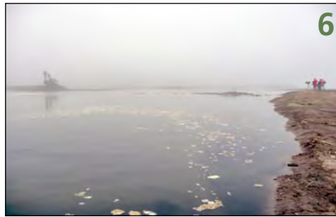
2 The double sill allows water to enter the slough gradually to equalize with interior water levels. Turbidity dissipates inside the restored site before exiting back out into the slough.
