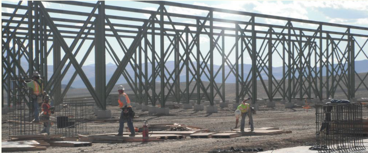
Construction workers at Ormat's McGinness Hills geothermal plant in Lander County.
