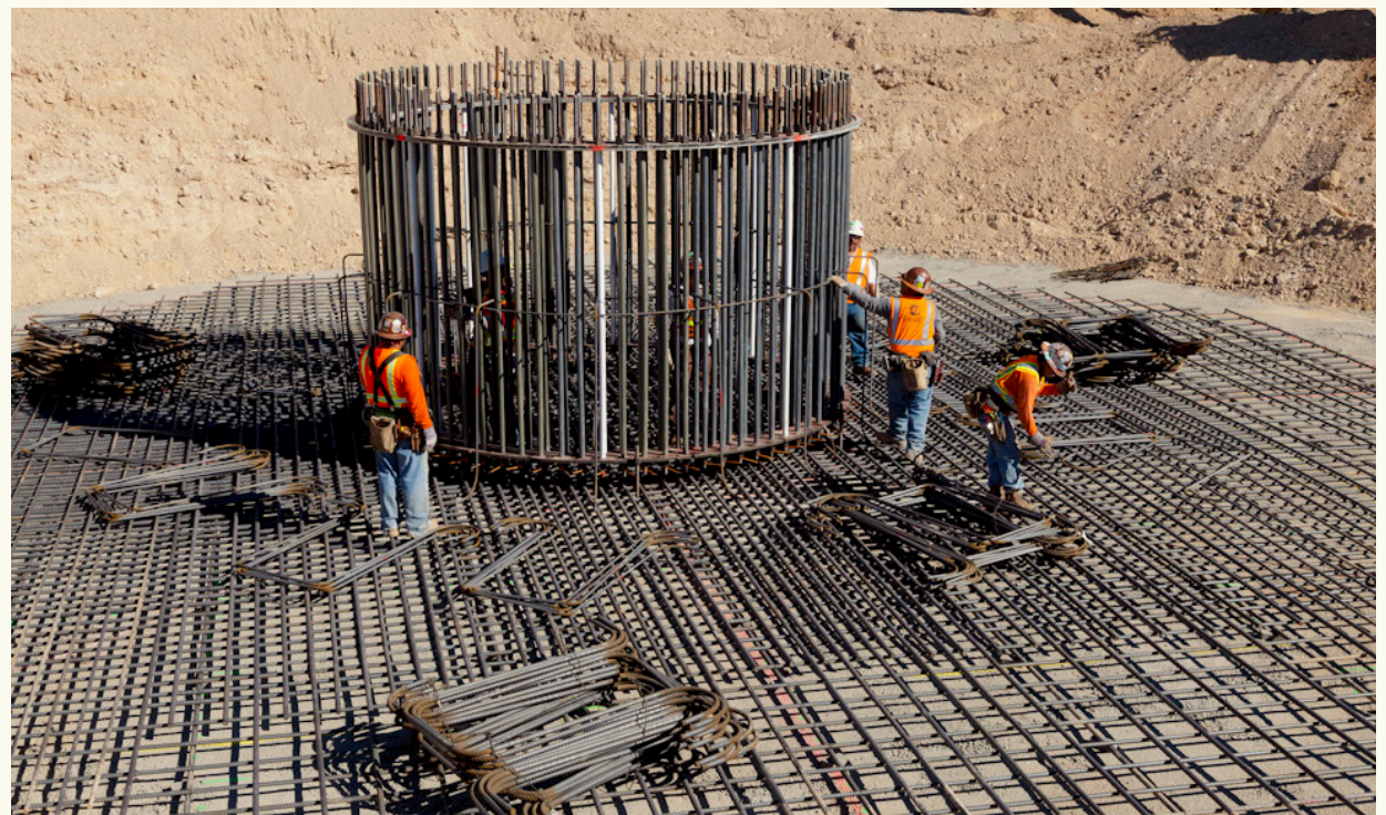
Wind turbine foundation construction at the Spring Valley project near Ely.
