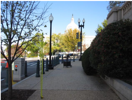
Protruding Tree Branch Creating Barrier
