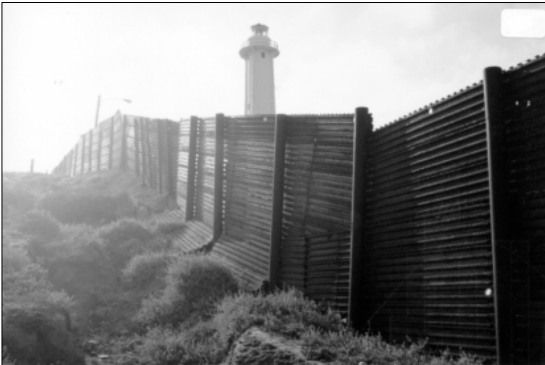
Figure B.3. Landing mat fence extends up the beach to a chain link fence.
