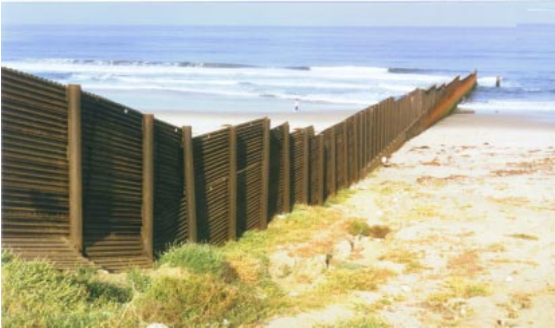
Figure 1. Landing mat design barrier.
