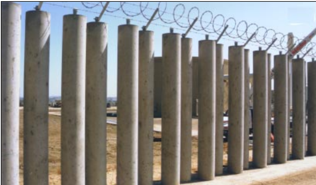
Figure 2. Bare bollard design barrier.
