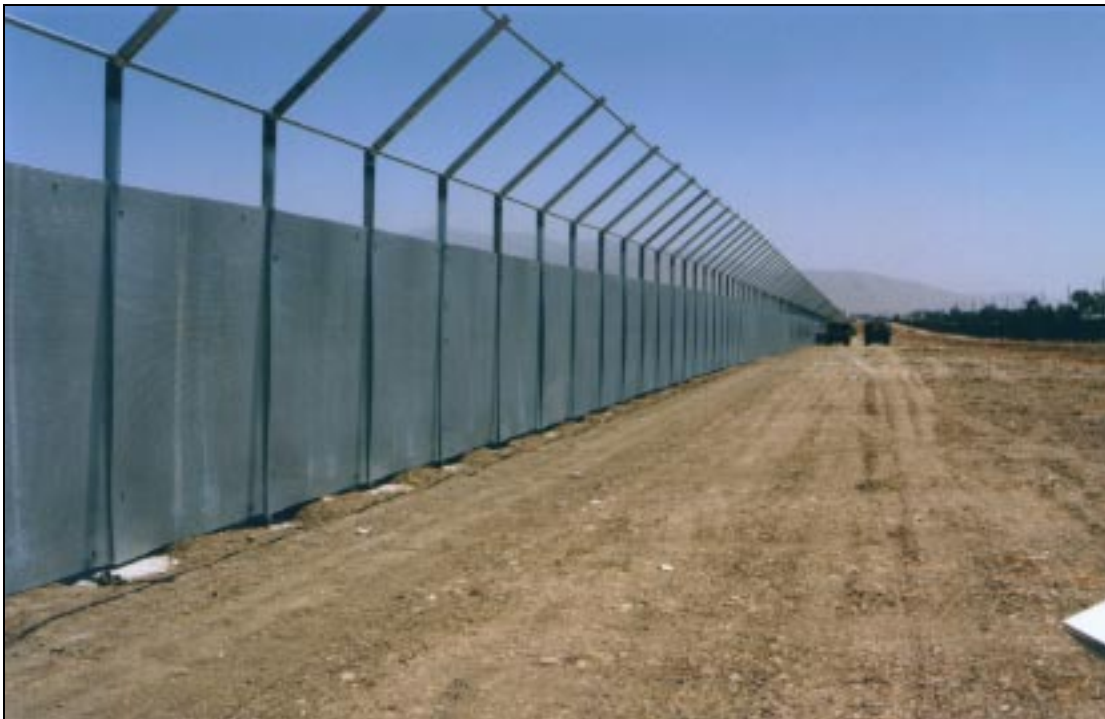
Figure 3. Sandia Fence design barrier.
