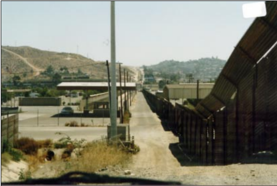
Figure B.17. Fence from the Tijuana levee through the former truck entry point to the border entry point.
