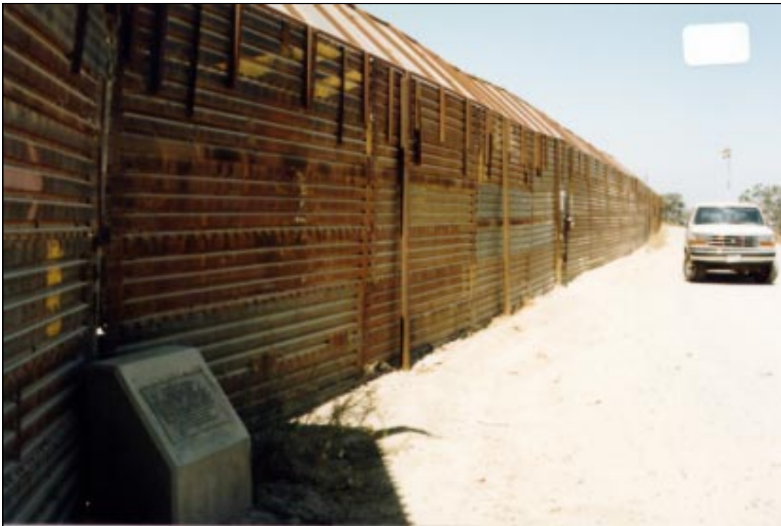
Figure B.16. Fence along the Tijuana levee.
