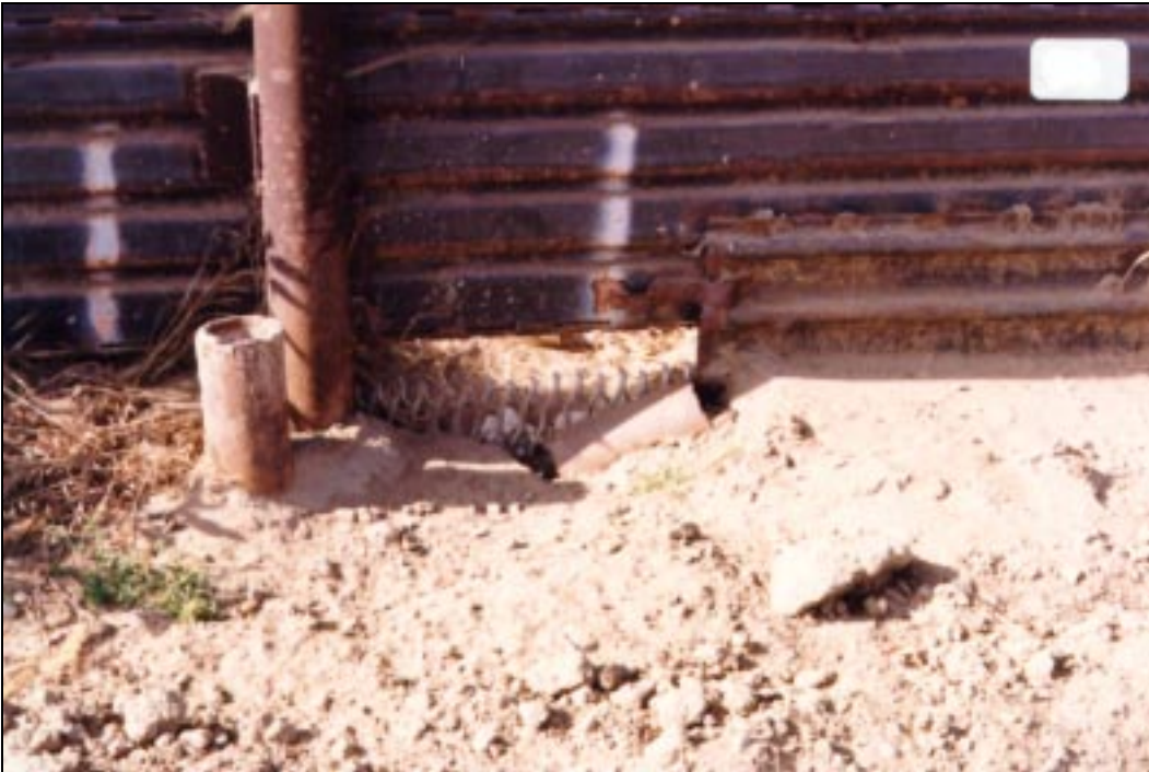
Figure B.9. Dig-under and cut pipe repairs 1,000 ft inland.
