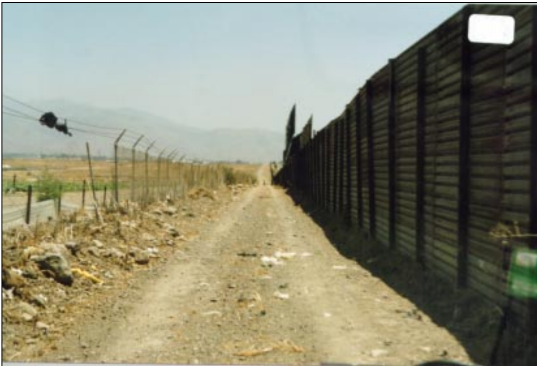
Figure B.22. Looking east along the fence toward the Otay hills.
