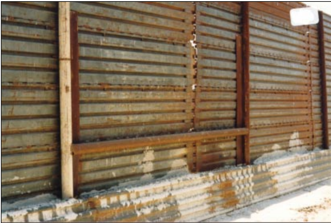
Figure B.24. Repairs to fence damaged by cutting and disassembly.
