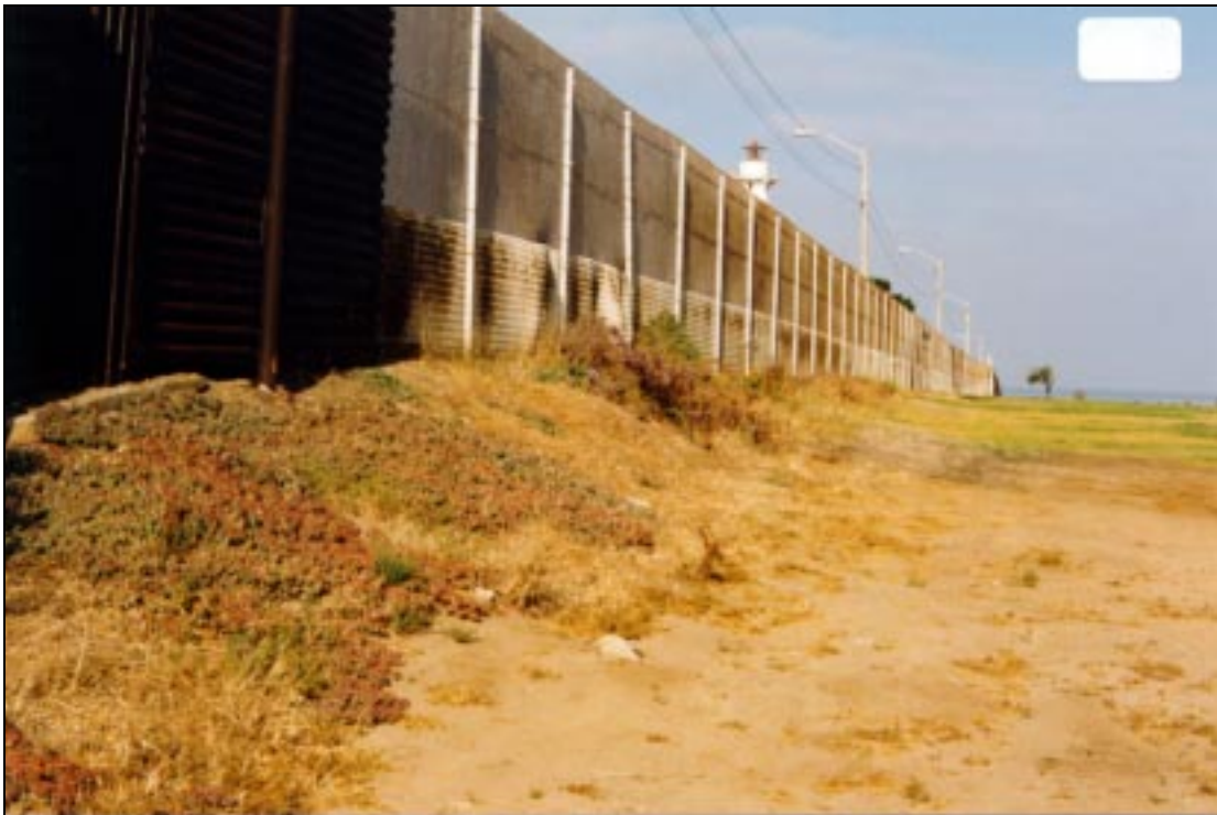
Figure B.5. Chain link fence connects the ocean fence and the first inland section of landing mat fence.
