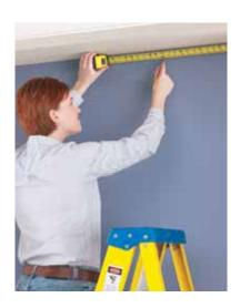
Mark the location of the studs on the wall. The easiest way to do this is with a stud finder. You can also knock on the wall with your knuckles and listen for spots where the wall no longer sounds hollow. Once you've located the first stud, measure to find the rest—the center of one stud will be 16 or 24 inches from the center of the neighboring studs.
