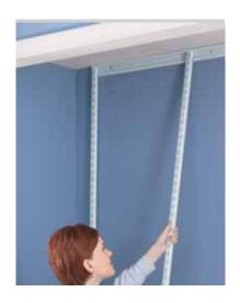
Hang the shelf standards from the track. Generally speaking, the standards should be no more than 24 inches apart, though manufacturer's recommendations may vary. Wherever possible, put each standard directly over a stud so you can screw directly into it. Verify that the standard is plumb and draw a line along it before screwing it in place. Screw it in place along the line, using the screws the manufacturer recommends.
