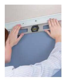
Make certain the hang track is level before driving the rest of the screws. If the ceiling is out of level, it may interfere with leveling the track. If so, drop the entire track 1/2 inch and reinstall.
