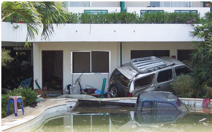
Figure 11. Destruction in Phuket, Thailand from the 2004 Indian Ocean Tsunami (Credit: NOAA/NWS/WCATWC)
