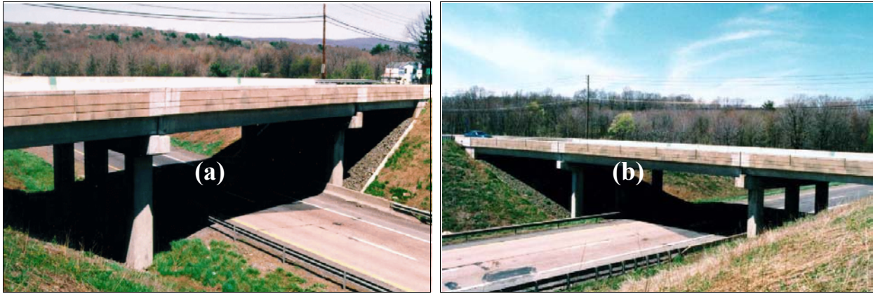
Figure 3-1. General views of the SR 2042 bridge structures over I-81: (a) west bridge and (b) east bridge.
