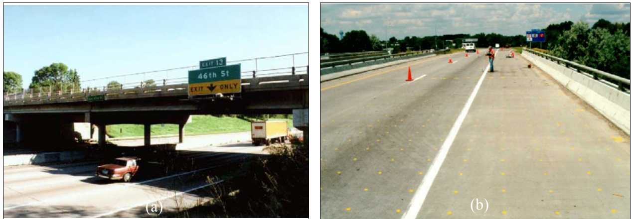
Figure 5-1. TH-3 over the Southview Boulevard bridge: (a) structure and (b) deck.
