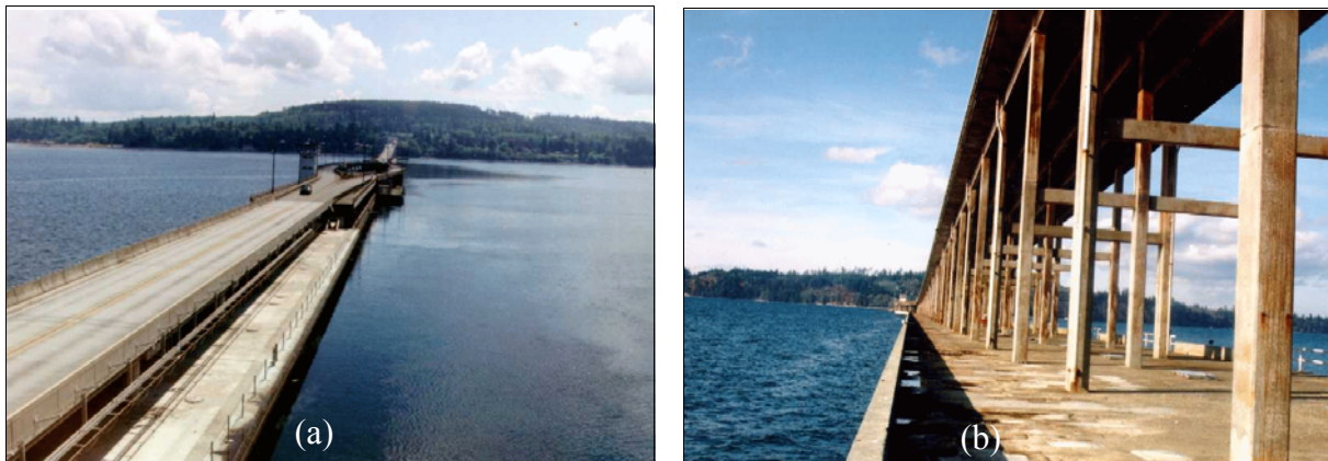
Figure 4-1. General views of the Hood Canal bridge.
