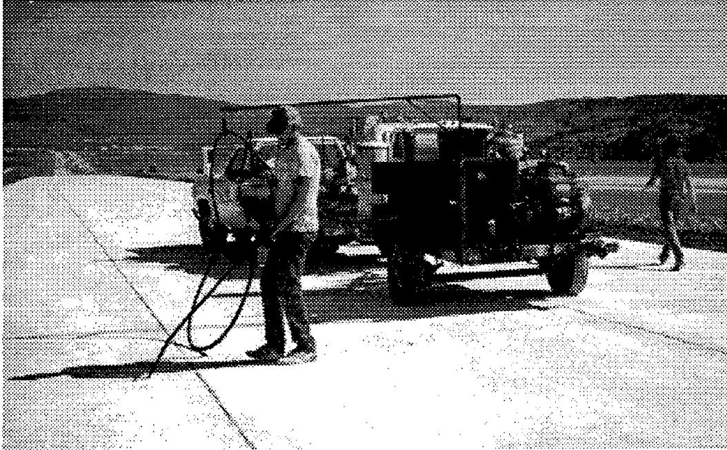
Figure 18. Hot-applied sealant installation at Heber City, Utah test site.
