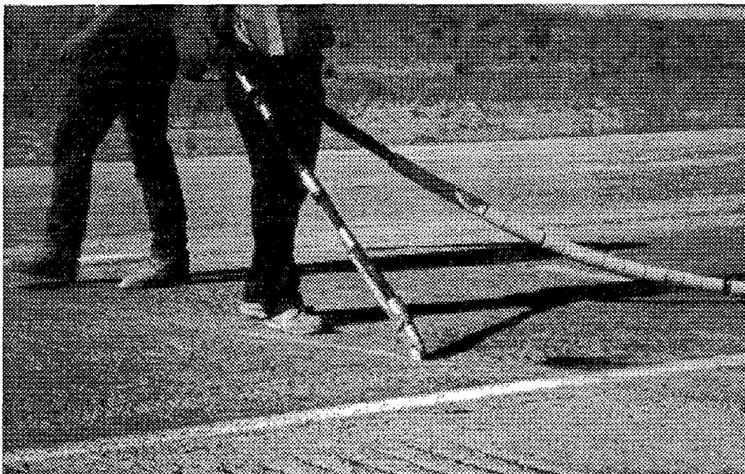
Figure 16. Sandblasting operation at Wells, Nevada test site.
