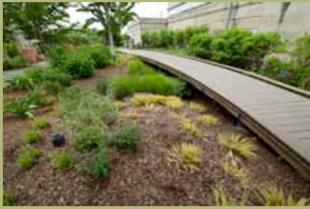
Rain gardens collect and infiltrate stormwater to help the AOC comply with requirements mandated within EISA2007 and the Clean Water Act.
