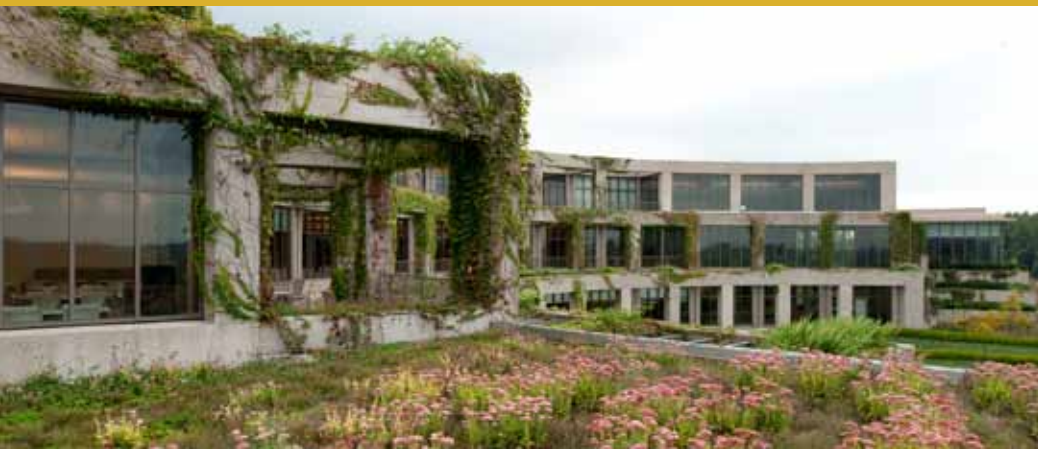
At left, the Library of Congress Packard Campus Green Roof. The building is covered with a 228,000 square foot extensive and intensive garden roof.
