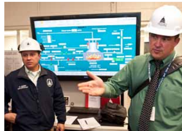
Employee of Sustainability and Energy Division works with the Power Plant team inside the control room.
