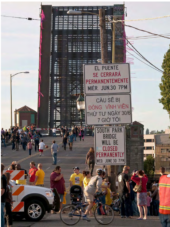
King CO, WA, is using TIGER grants to replace the closed South Park Bridge
