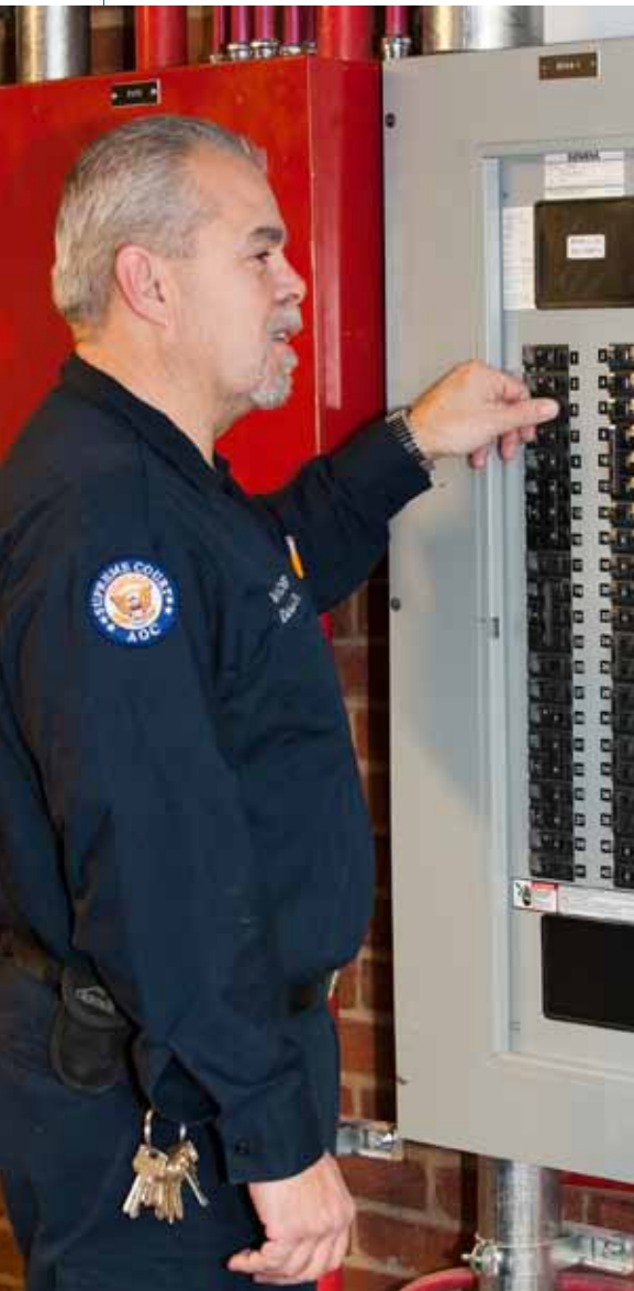
AOC electrician Mike Wilcher helps ensure that the powerful are powered.
