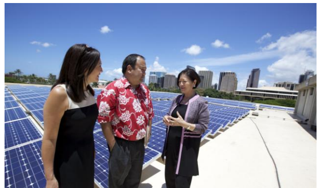
Congresswoman Hirono meets with Jan Gouveia and Dean Seki of the Hawaii Department of Accounting and General Services to learn more about the solar panels installed on the roof of the Kalanimoku Building.
