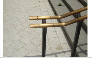
**Hazard**: Protruding handrails create projection hazard not compliant with 29 CFR § 1910.23(e)(5)(i), 2000 NFPA 101 7.2.2.4.5, ANSI/ASSE A1264.1-2007 Section 5.8 and ASTM E 985-00 Section 4.3.2.
