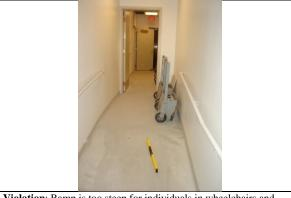
**Violation**: Ramp is too steep for individuals in wheelchairs and does not comply with 28 CFR Part 36 Appendix A Section 4.8.2. **Solution**: Regrade ramp equal to or less than 8.3% grade.
