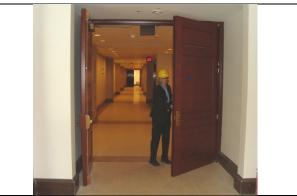
**Hazard**: Door swings against direction of egress travel, which does not comply with 2000 NFPA 101 7.2.1.4.2. **Solution**: Rehang door to swing in the direction of egress travel.
