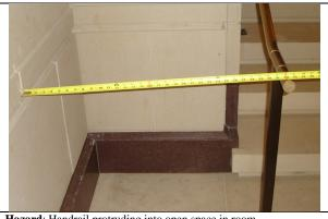
**Hazard**: Handrail protruding into open space in room. **Solution**: End handrail at bottom riser and make compliant with 29 CFR § 1910.23(e)(5)(i), 2000 NFPA 101 7.2.2.4.5, ANSI/ASSE A1264.1-2007 Section 5.8 and ASTM E 985-00 Section 4.3.2.
