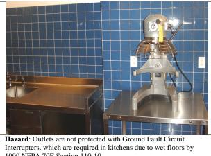
1999 NFPA 70E Section 110-10. **Solution:** Install low cost GFCI outlets in the kitchen and near all water sources.
