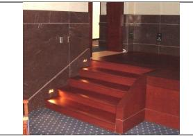
**Hazard**: Stairway with greater than 4 risers has no handrails, not complying with 29 CFR § 1910.23(d)(1). **Solution**: Install handrails compliant with 29 CFR § 1910.23(d)(1).
