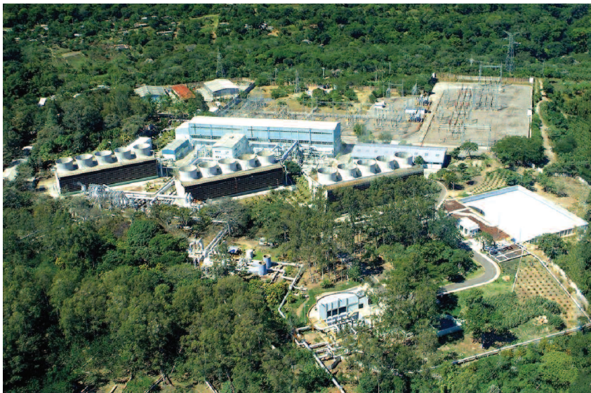
Figure 8.3 Ahuachapan geothermal facility after revegetation, circa 2005 (LaGeo, 2005).
