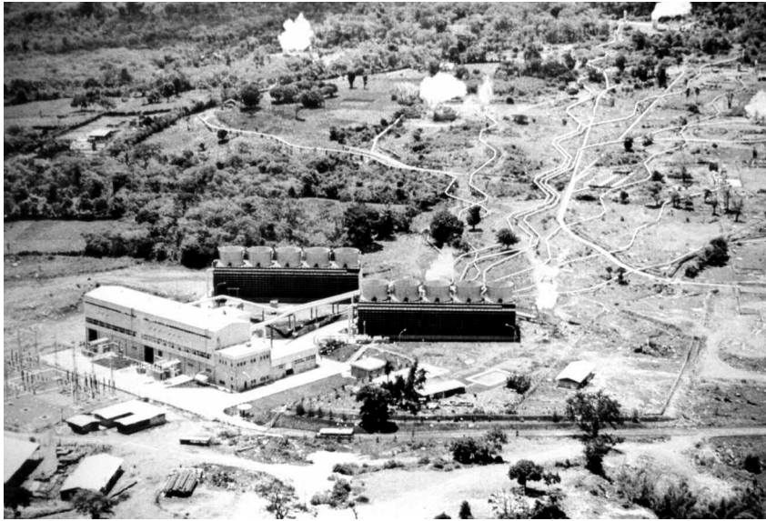
Figure 8.2 Ahuachapan geothermal facility after commissioning around 1977 (DiPippo, 1978).
