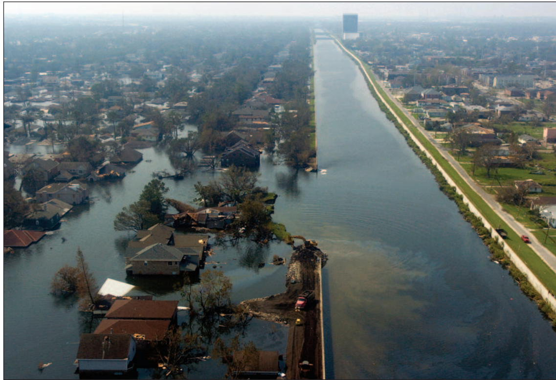
A canal breached, New Orleans
