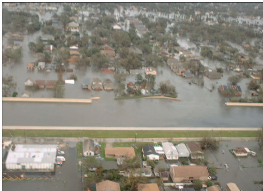
Breached floodwall, New Orleans Marty Bahamonde photo
