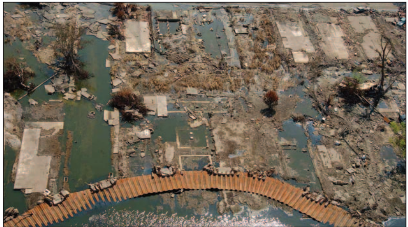
Ripped-out sheetpile with chunks of floodwall attached, New Orleans Louisiana National Guard photo
