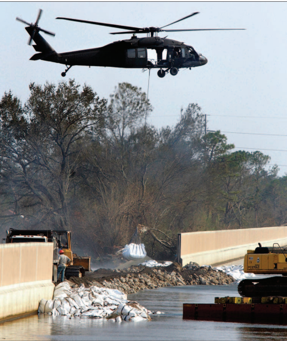
Plugging a breached floodwall, New Orleans
