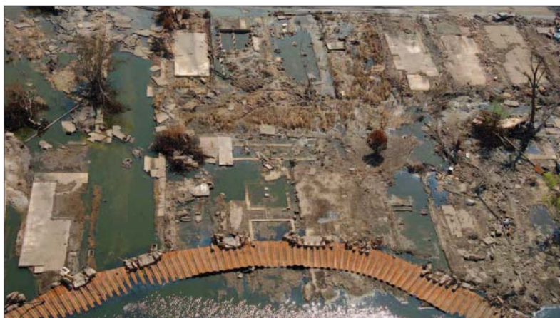
Ripped-out sheetpile with chunks of floodwall attached, New Orleans Louisiana National Guard photo
