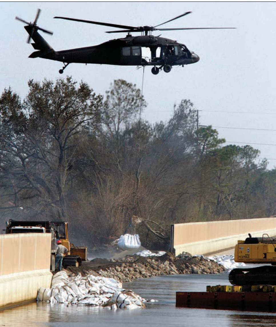
Plugging a breached floodwall, New Orleans
