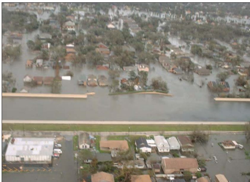
Breached floodwall, New Orleans Marty Bahamonde photo
