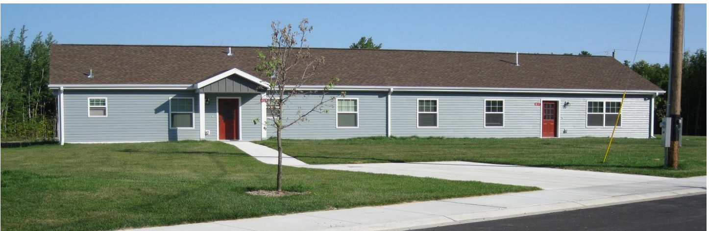
A building at the New Moon development
