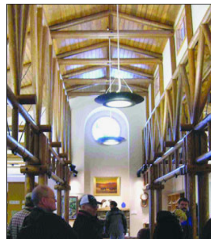
Innovative small-diameter wood trusses for the library in Darby, MT.
