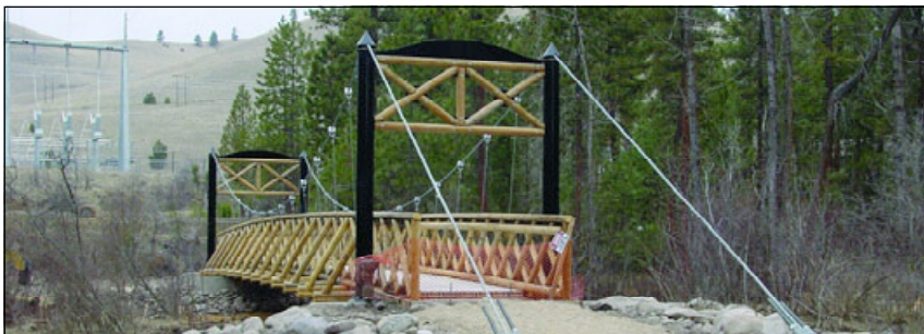
Small-diameter-wood bridge near Missoula, MT.
