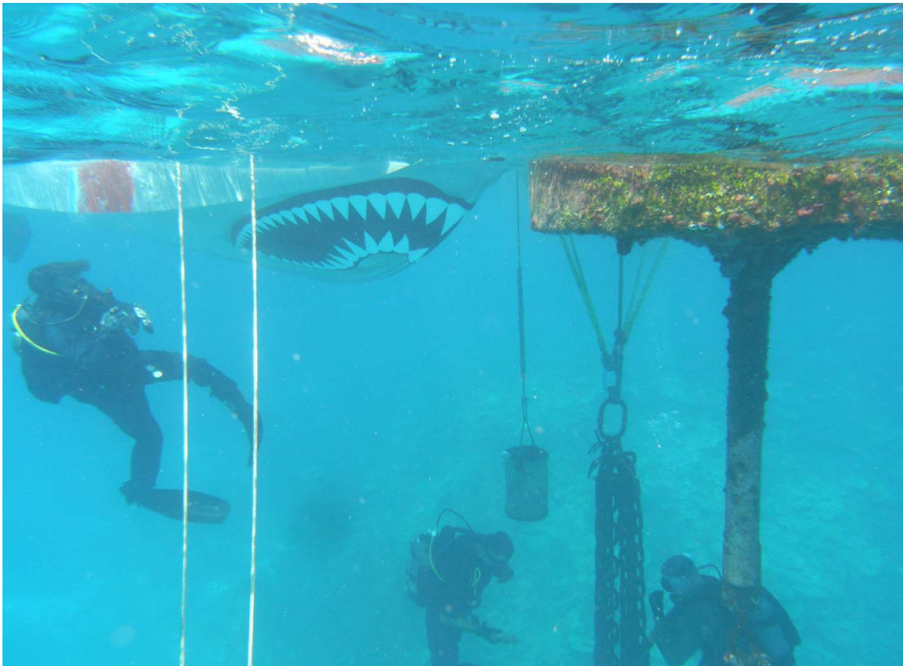
USCGC SEQUOIA's (WLB- 215) ATON dive team conducts a subsurface mooring inspection and chain replacement in Kwajalein Atoll, Republic of the Marshall Islands. Photo by BOSN Joe Toth.
