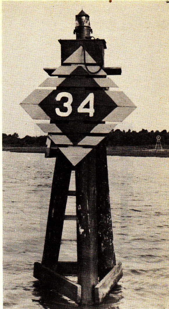
FIGURE 24-53.—Three-pile dolphin (Fifth District).
