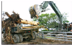
Dozers, Scrapers, Loaders, Excavators, Dump Trucks
