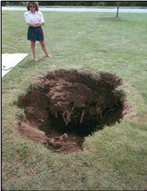
Figure 7. Karst-related hazards often take the form of collapse sinkholes, such as this example from a residential area in Jessamine County, Kentucky.
